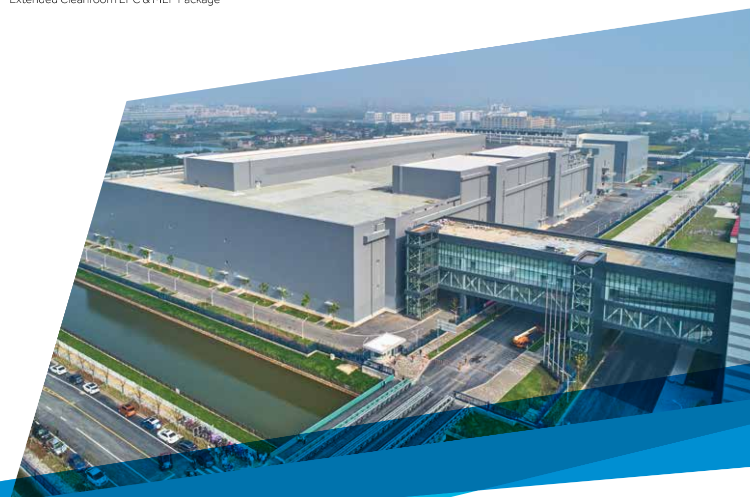
HLMC 300mm Wafer Fab Shanghai, China 2016 - 2018 Extended Cleanroom EPC & MEP Package
