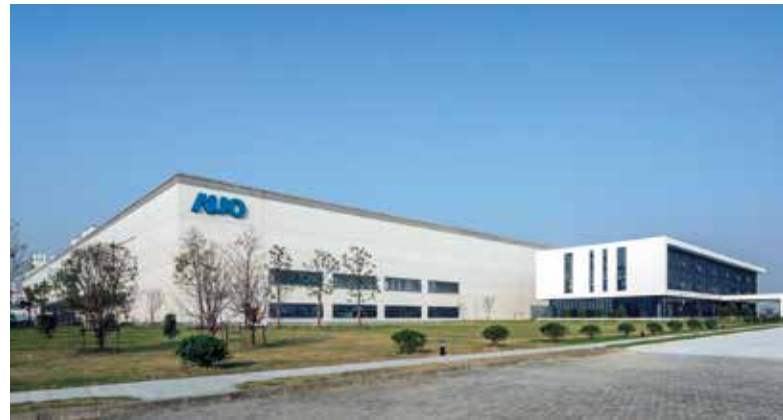
AUO TFT Display Facility Kunshan, China 2015 - 2017 Extended Cleanroom EPC
